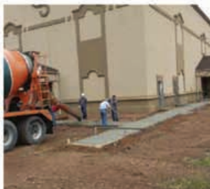
Above: Pouring concrete for sidewalks. Right: Pipes for fire suppression system.
